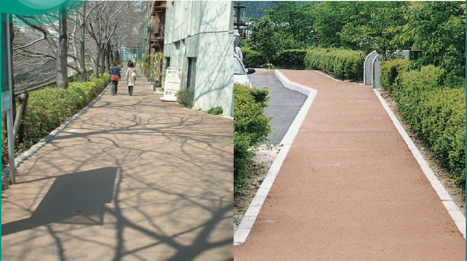
**This is a natural-colored landscaping pavement that sprays a thin layer of special aggregate onto road surfaces.**
